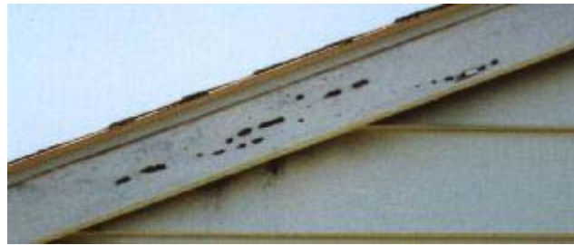
Figure 10. Woodpecker damage due to foraging for carpenter bee larva on fascia boards of a house
